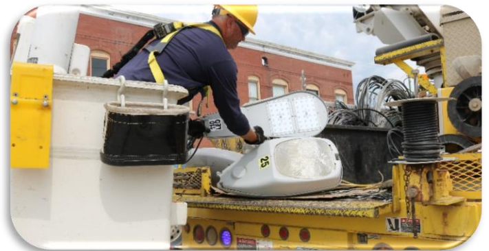
SCPPD Lineman, Matt Hoferer, holds a new LED fixture next to the previous HPS street light.
